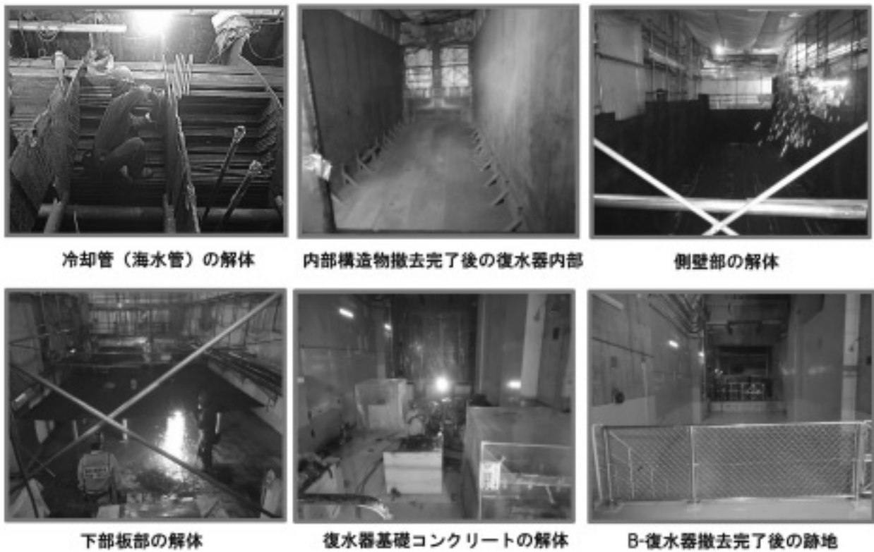
Fig. 7 Examples of dismantling performance in condenser
